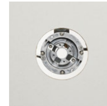
Install the drywall.
