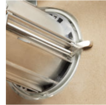
Screw mud plate and junction box to the wall. Junction box will grip the interior wall with two wing brackets.
