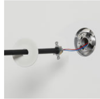
Connect fixture to junction box.
