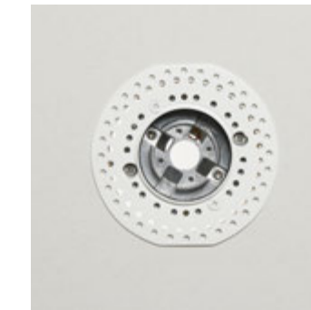
Install the mud plate.
