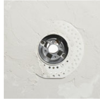
Mud the wall and plate.
