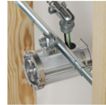
Connect power from conduit to junction box.
