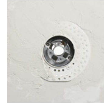
Mud the wall and plate.
